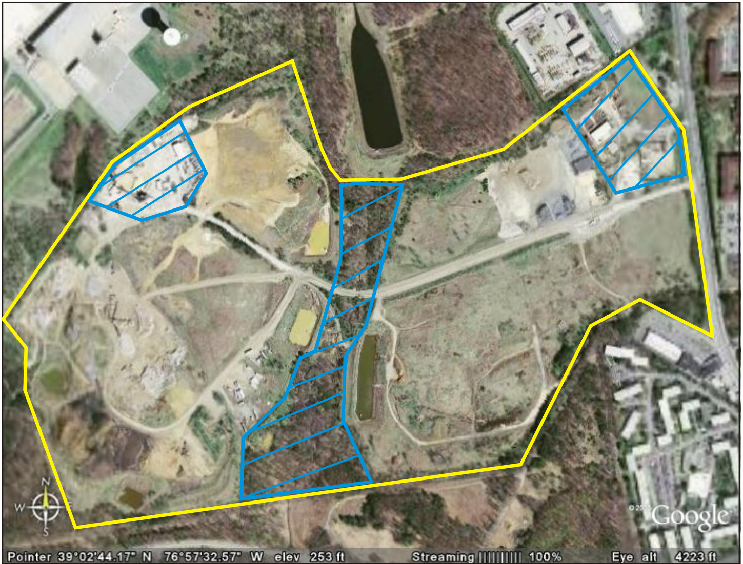
MINED AND RECLAIMED AREAS OF SITE (Unmined areas outlined in blue)
