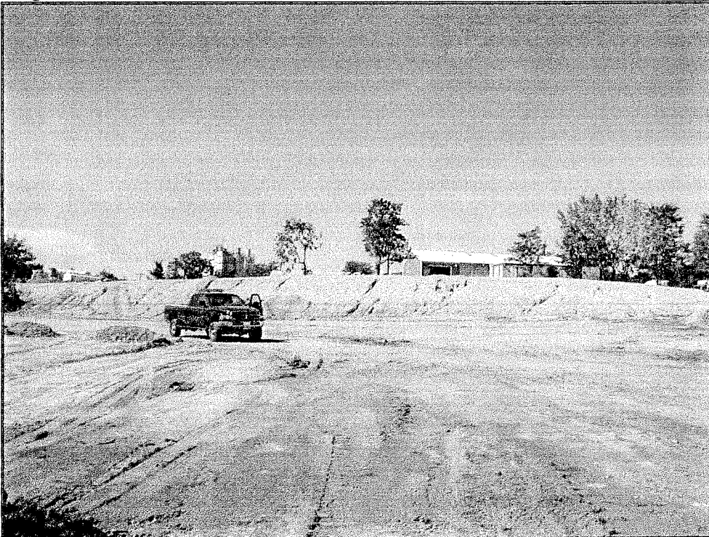
Photograph #2 – As mining operations are completed, areas are now being reclaimed with controlled fill materials including soil, asphalt, and concrete.
