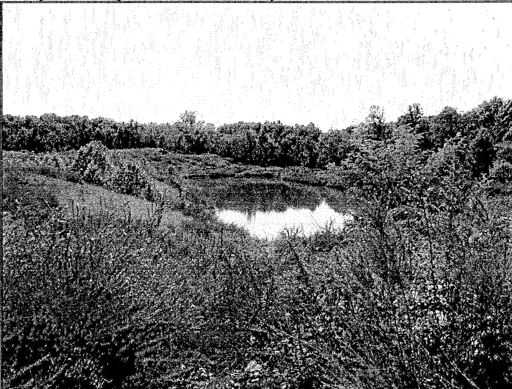
Photograph #6 – One of the six sediment basins located on site to filter stormwater runoff across the subject property.
